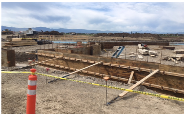
Foundation Wall Form Work
