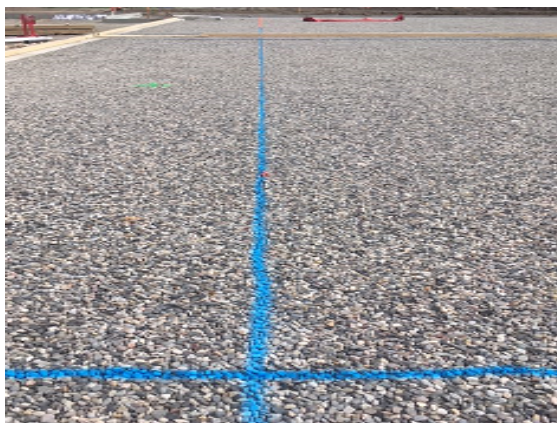
Layout for Excavation
