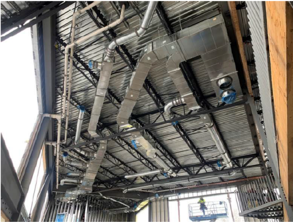
Figure 07: Ductwork in Building 2A
