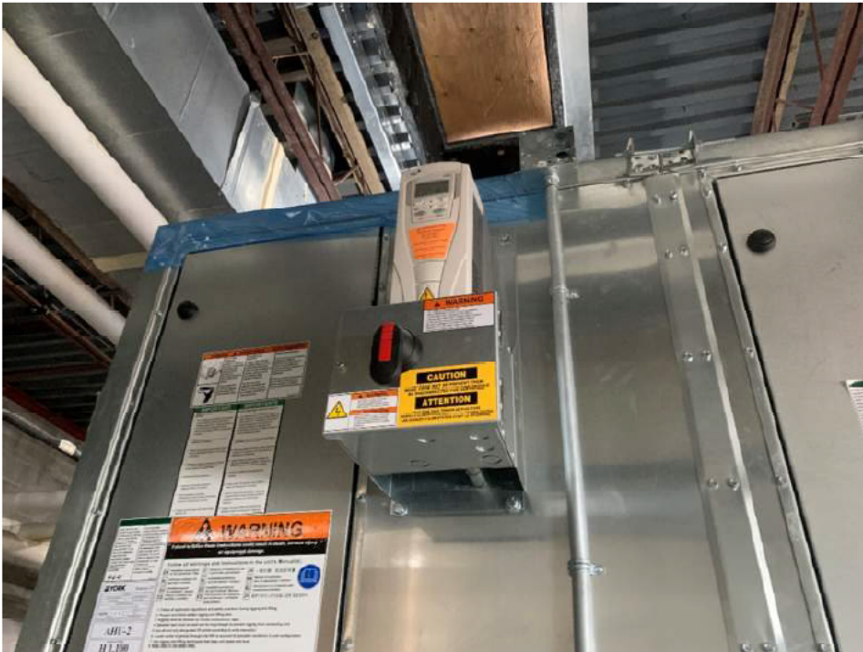
Figure 03: Cover ALL VFDs during construction.
