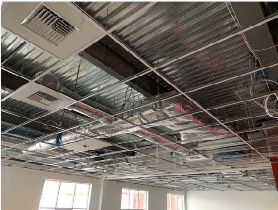
Figure 10: GRD install in Building 3B
