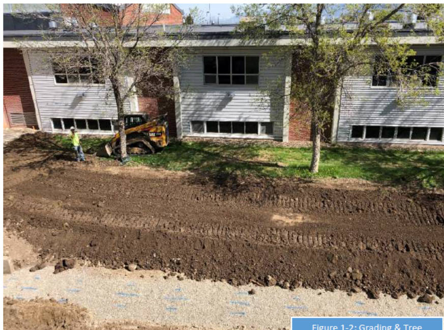
Figure 1-2: Grading & Tree Protection Deficiency
