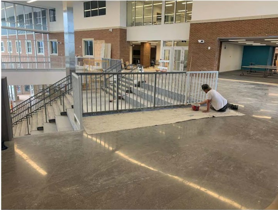
Figure 03: Painting the commons guardrails
