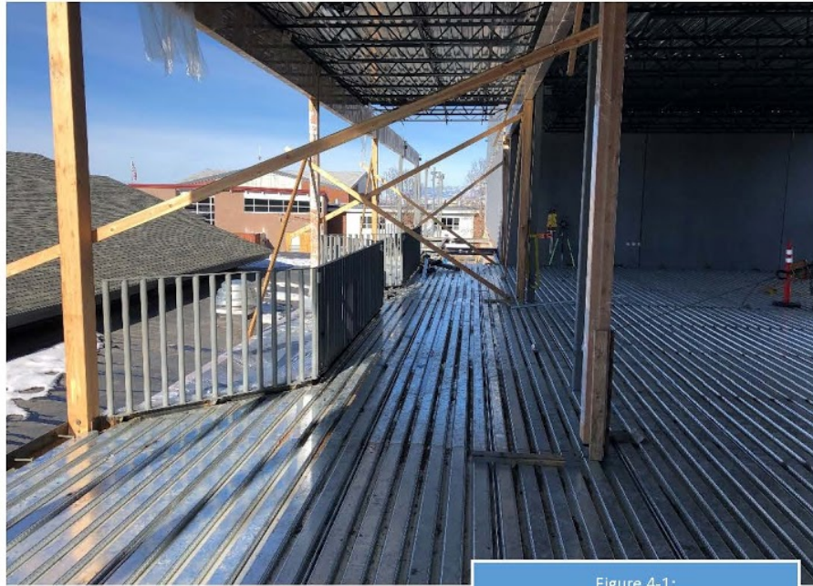
Figure 4-1: Floor Opening Railings
