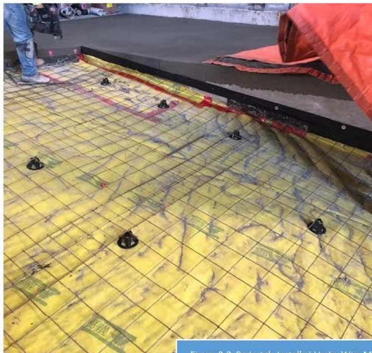
Figure 2-2: Pedestals Installed Under Wire Mesh
