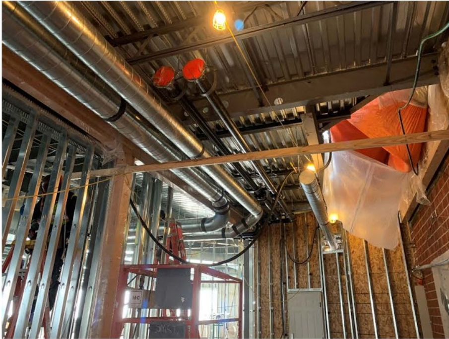
Figure 01: Ductwork and Hydronic Pipe in Building 3B.
