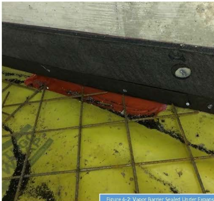
Figure 4-2: Vapor Barrier Sealed Under Expansion Joint
