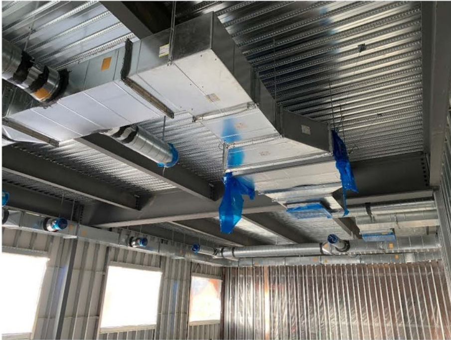
Figure 01: FCU install in 3B
