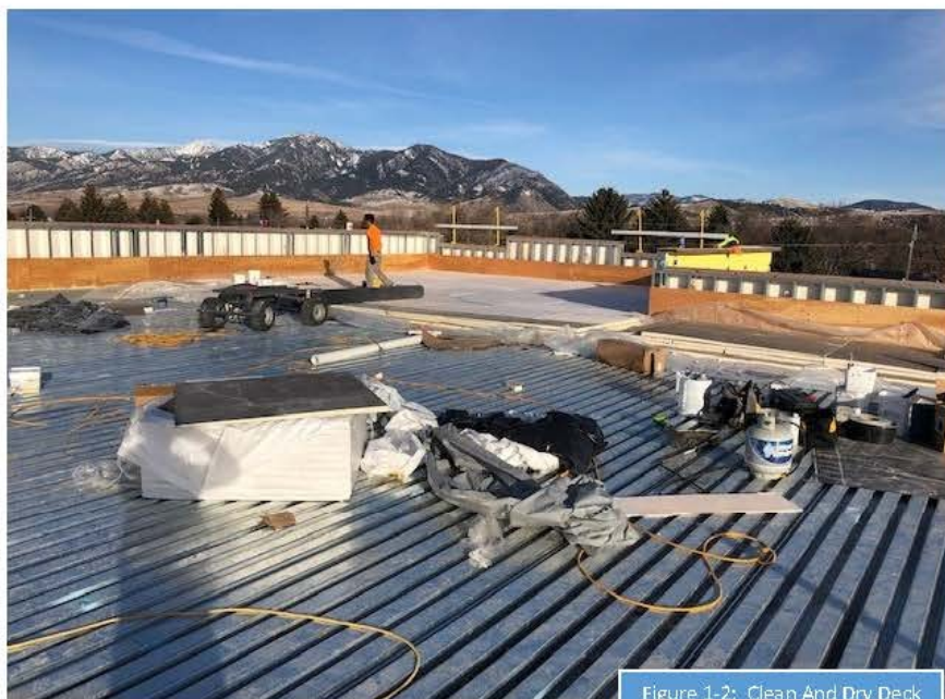
Figure 1-2: Clean And Dry Deck With New Roof Installation
