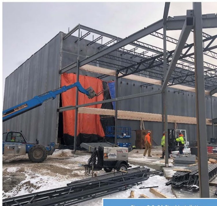
Figure 2-2: 2A Steel Installation
