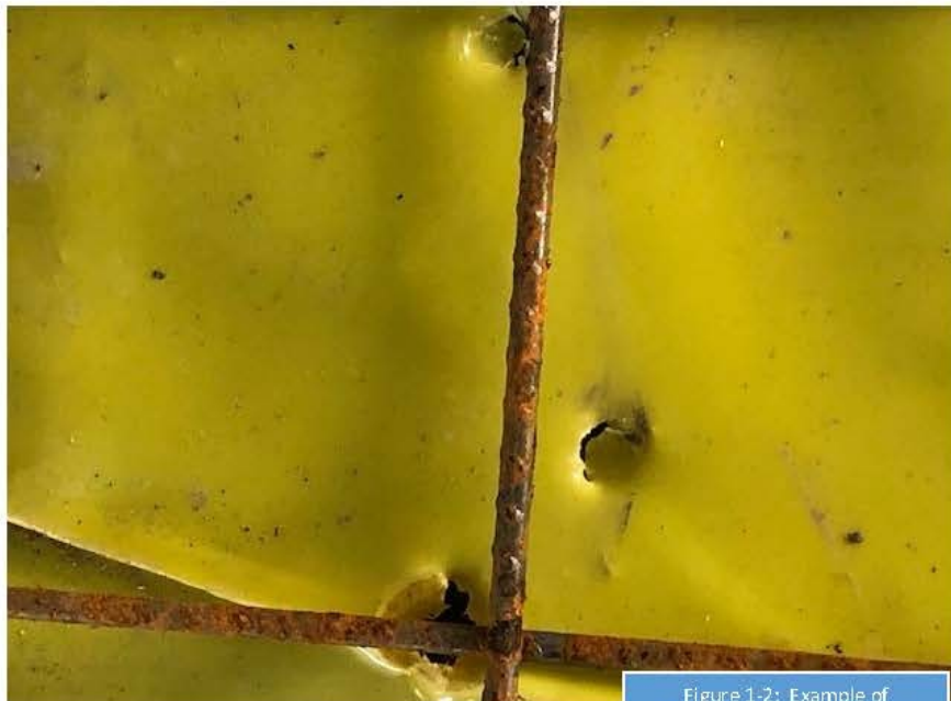
Figure 1-2: Example of Penetrations in Vapor Barrier
