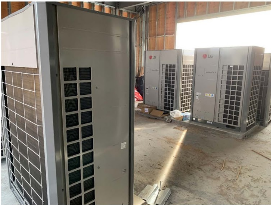
Figure 06: ACCU-2 and ACCU-3 in Penthouse.
