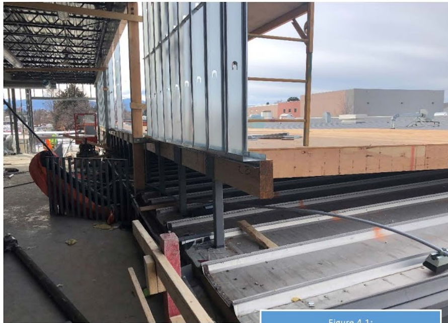
Figure 4-1: Building 3A Roof Overframe
