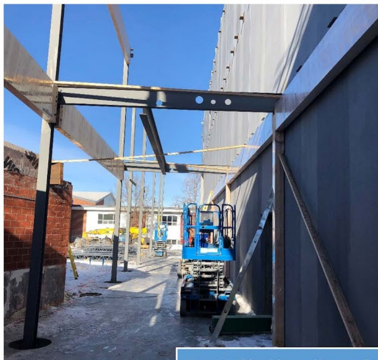
Figure 3-2: Glulam Column and Beam Installation
