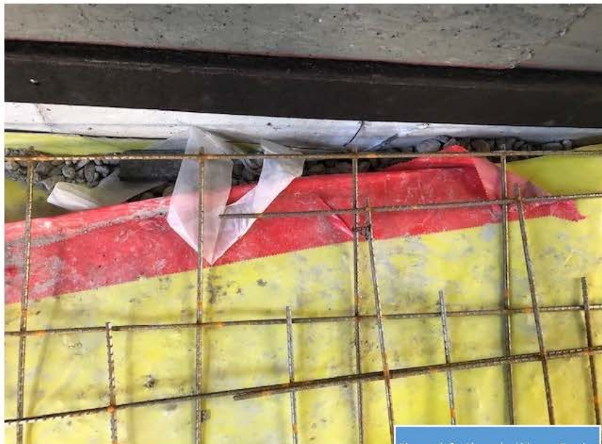
Figure 1-2: Unsealed Vapor Barrier
