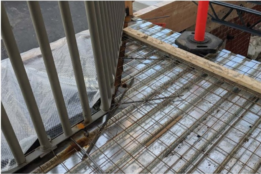
Image 3 : Diagonal bar at corner condition
