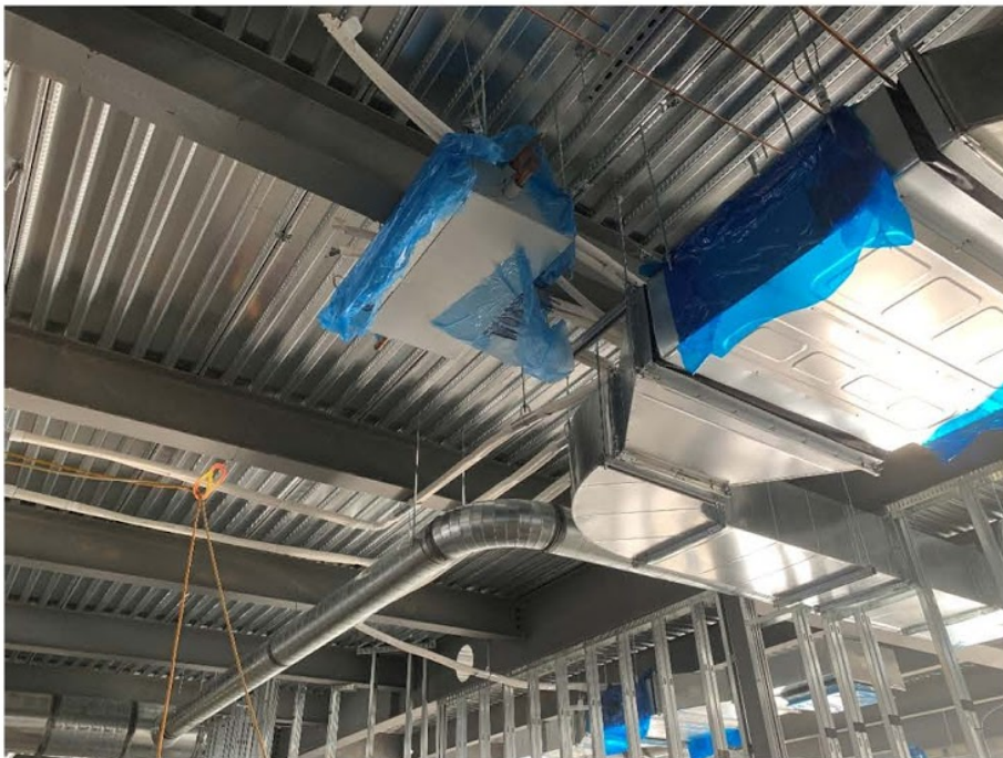
Figure 02: VRF HRB and Refrigerant Pipe.
