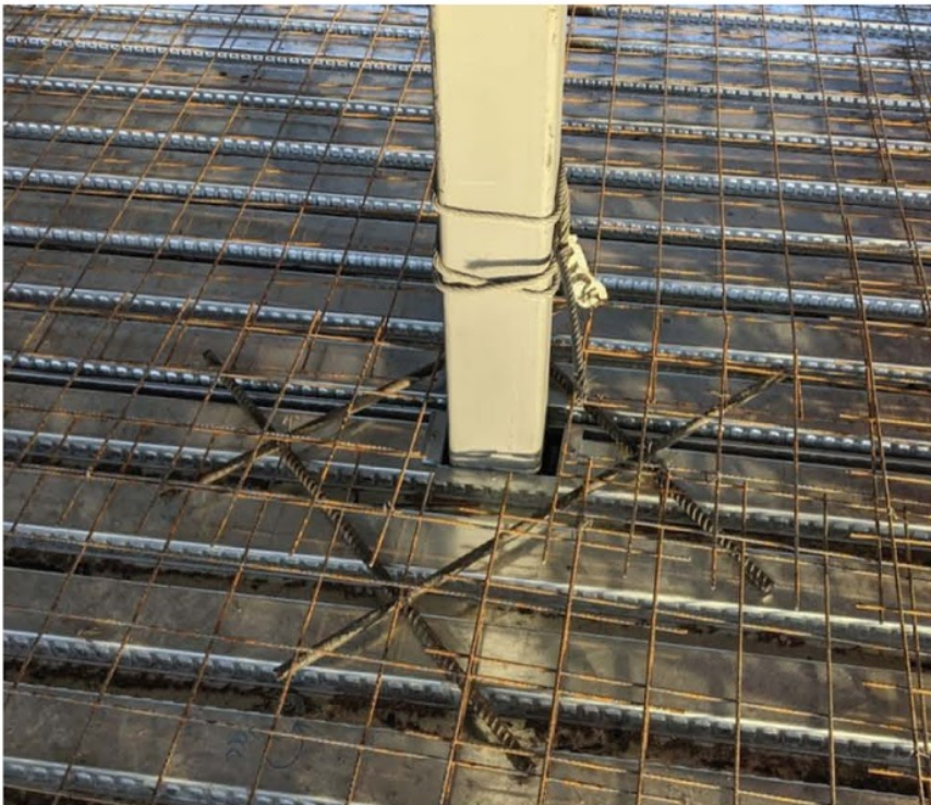
Image 4 : Diagonal bars at column condition
