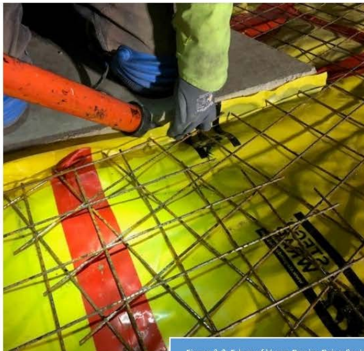
Figure 3-2: Edges of Vapor Barrier Being Sealed
