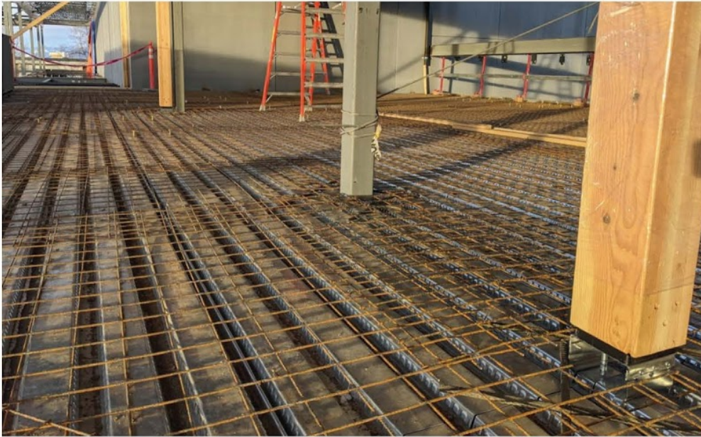
Image 1 : Welded wire reinforcing
