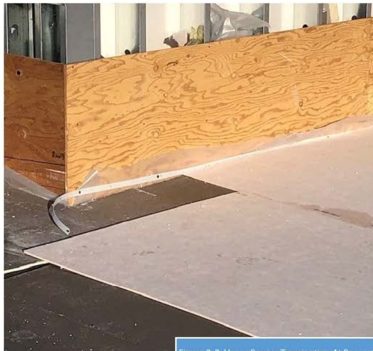
Figure 2-2: Vapor Barrier Termination At Parapet Wall
