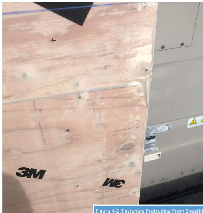
Figure 4-2: Fasteners Protruding From Sheathing Under Weather Barrier
