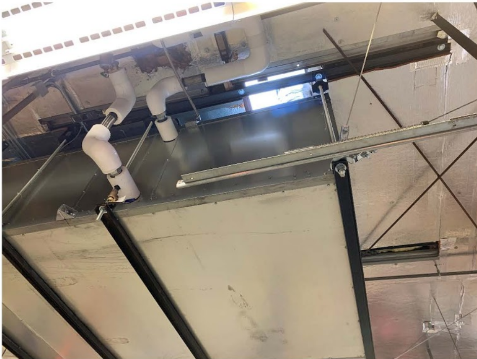
Figure 04: Roof penetration sealed with plastic
