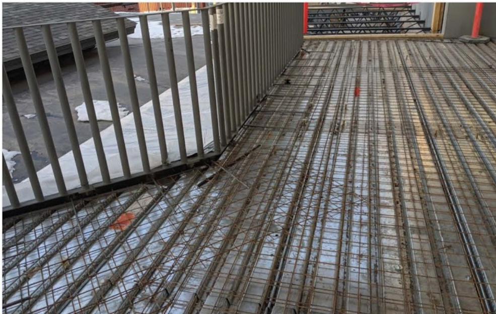
Image 2 : Welded wire reinforcing
