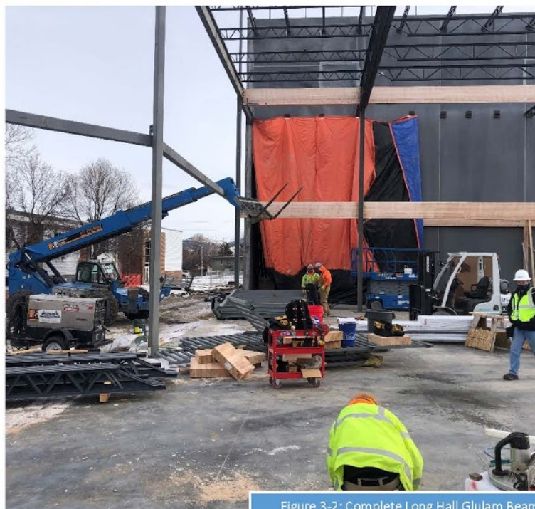
Figure 3-2: Complete Long Hall Glulam Beam Installation
