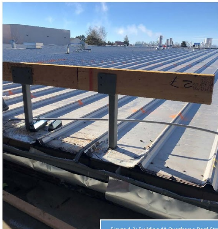
Figure 4-2: Building 4A Overframe Roof Structure
