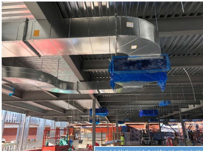
Figure 3-2: Mechanical duct and fan coil units in building 3B
