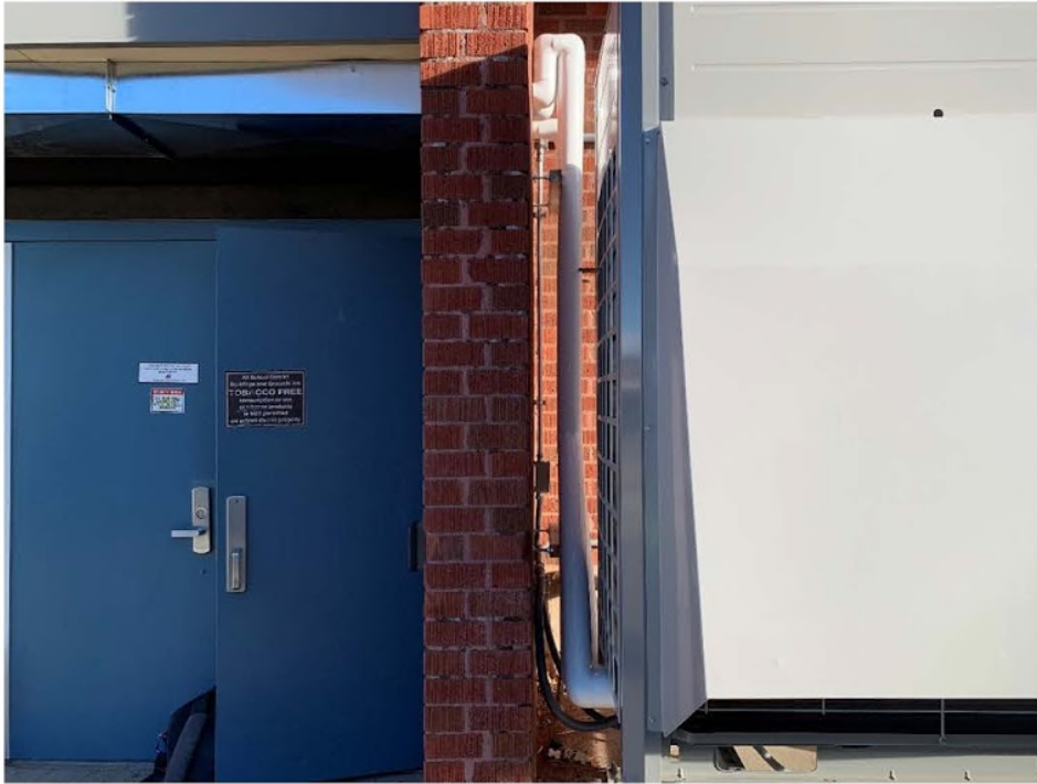
Figure 03: VRF Pipe Insulation complete.
