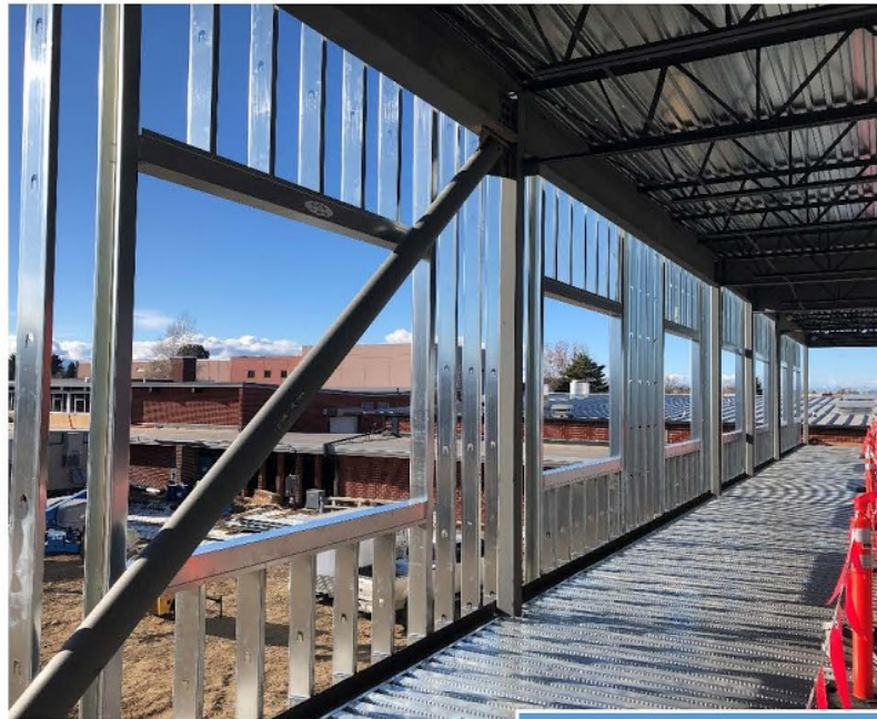
Figure 1-1: Building 3B exterior wall framing
