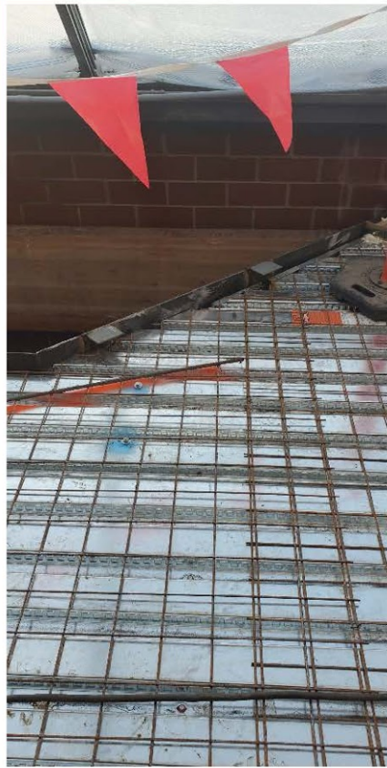
Image 4: Typical handrail attachment embed
