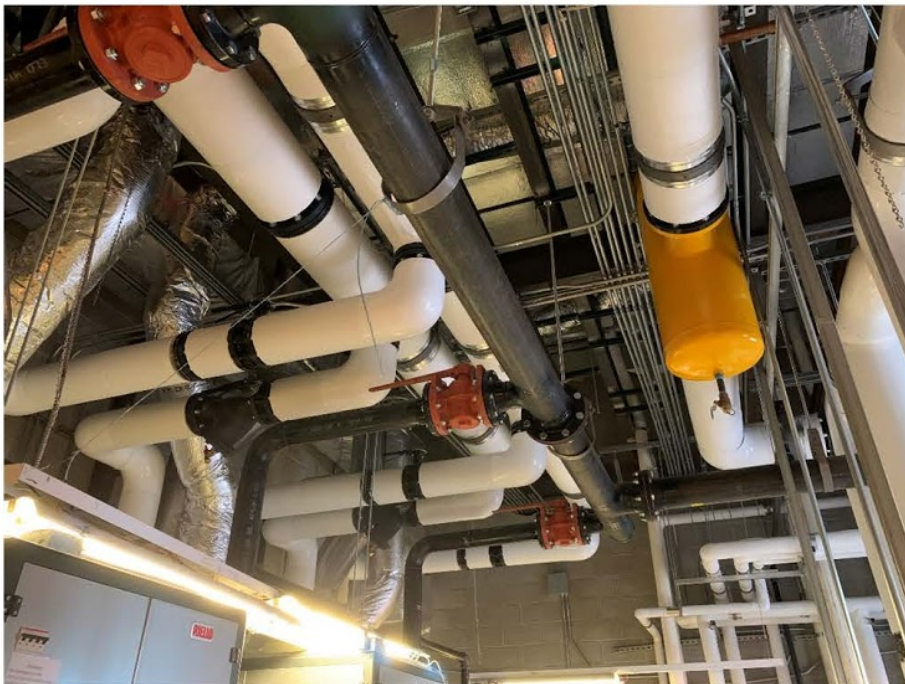
Figure 02: H-Wing Boiler Room Insulation
