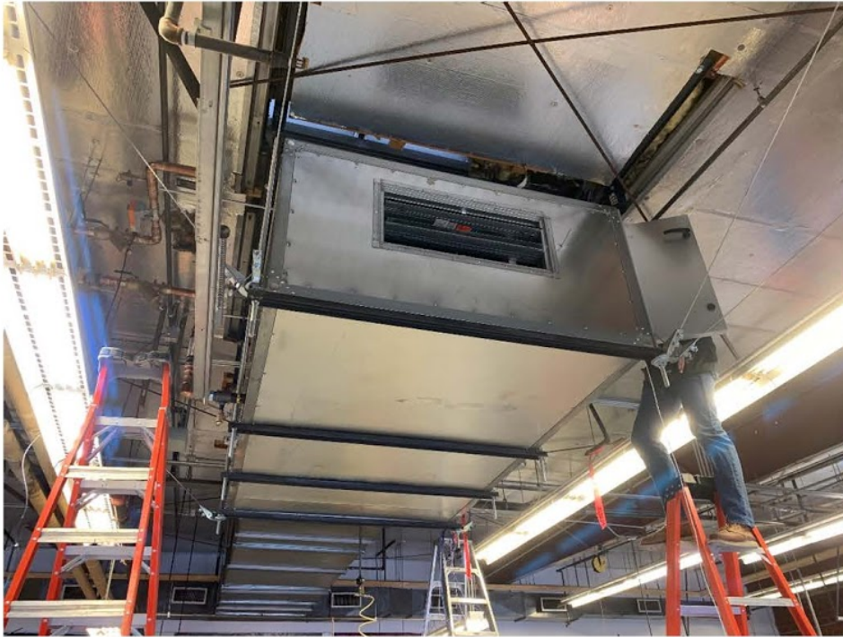
Figure 03: AHU-5 installation in the Auto Shop
