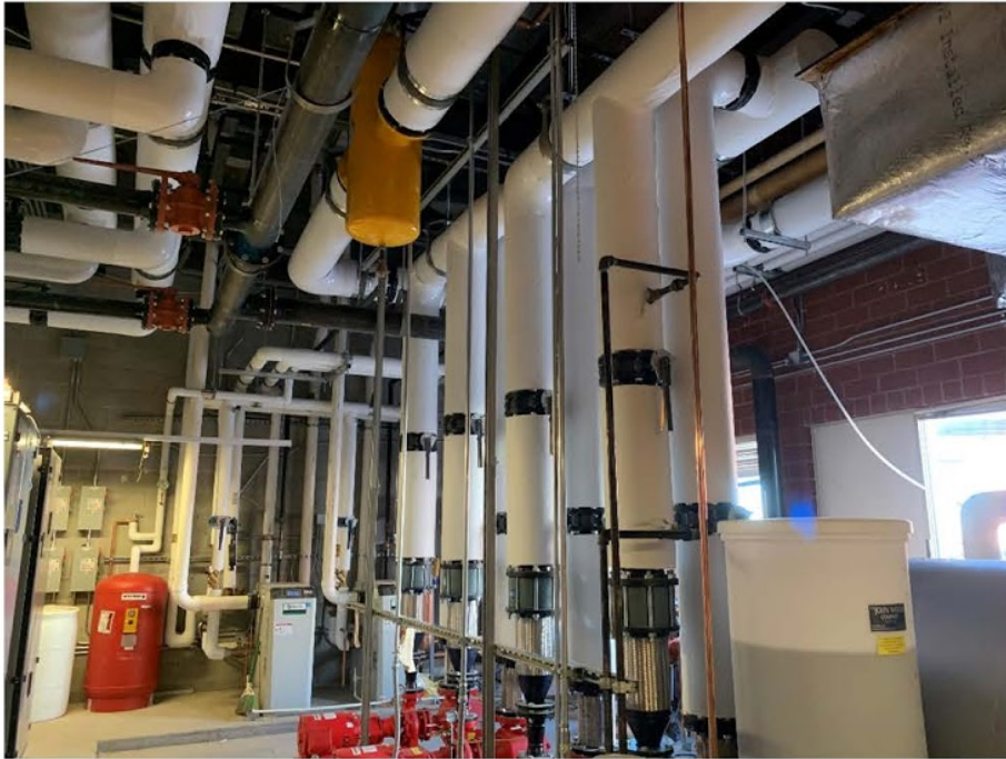
Figure 01: H-Wing Boiler Room Insulation
