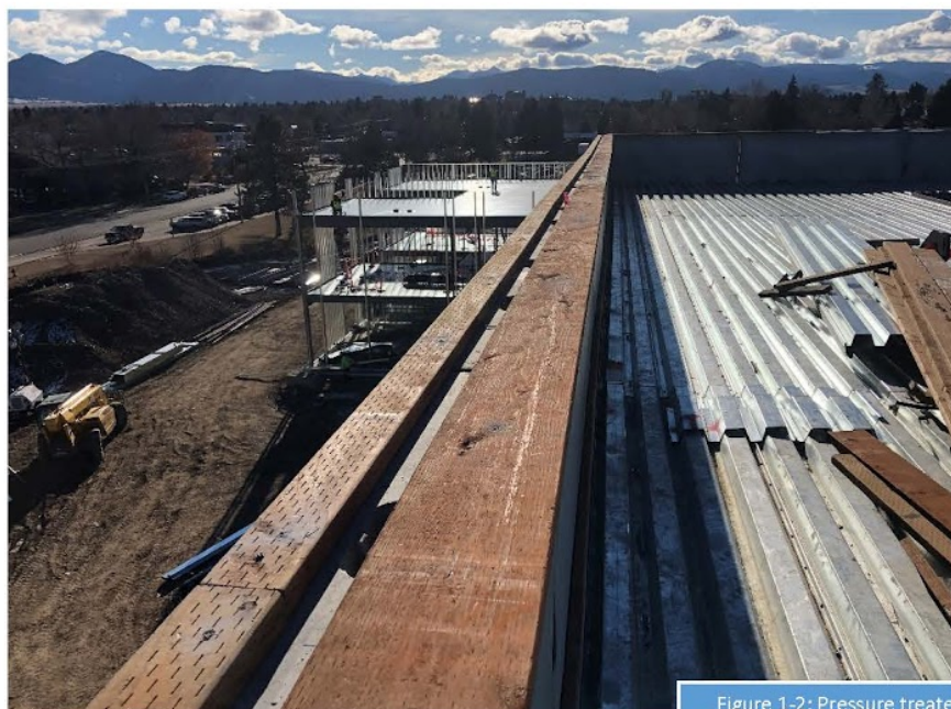
Figure 1-2: Pressure treated lumber at auditorium roof parapet
