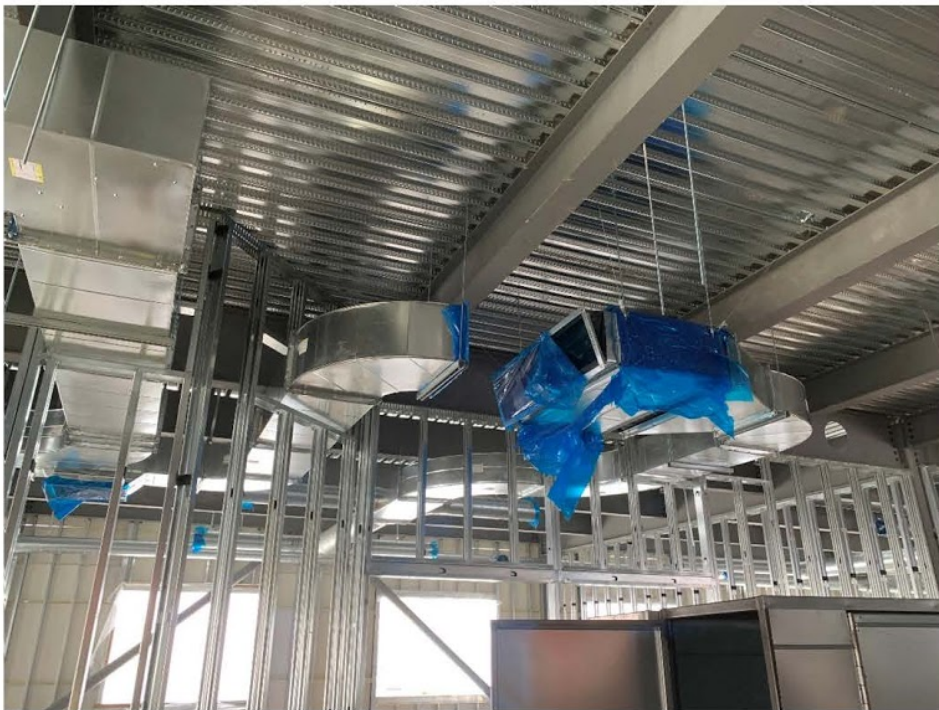
Figure 06: Cover all ductwork and equipment in place
