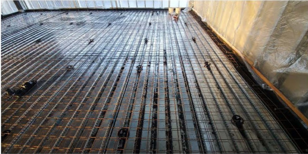
Image 1: Typical chaired reinforcement
