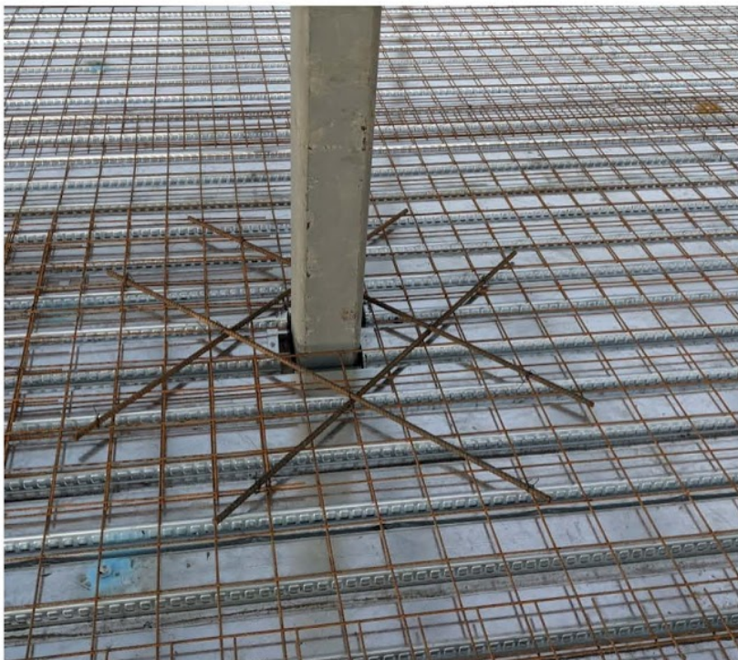
Figure 4: Rebar dowels around steel column
