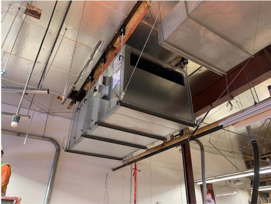
Figure 01: AHU-4 install in the wood shop
