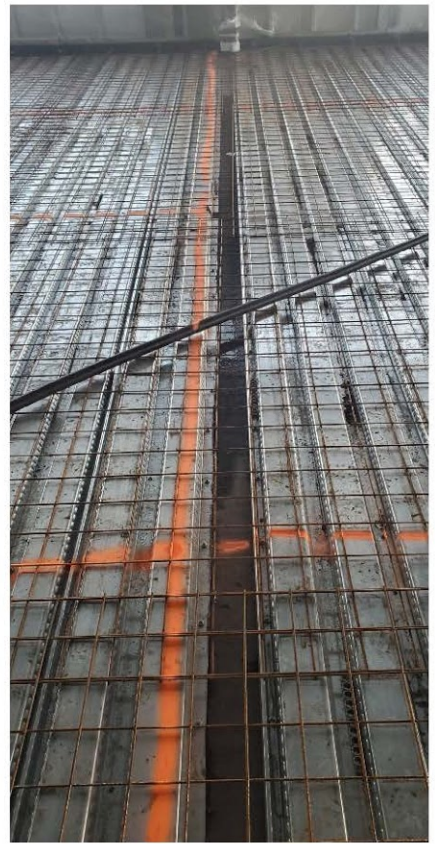
Image 6: Steel girder missing headed studs
