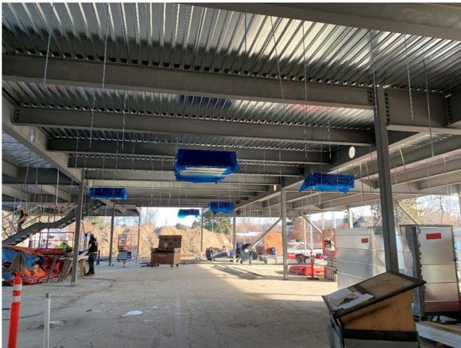
Figure 04: VRF FCU Installation in Building 3B.
