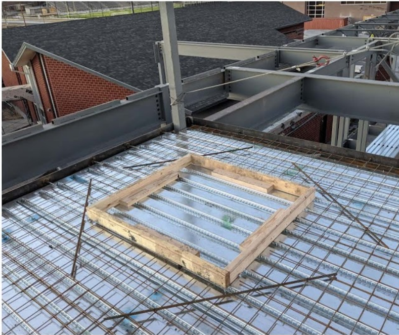
Figure 3: Rebar dowels around slab opening
