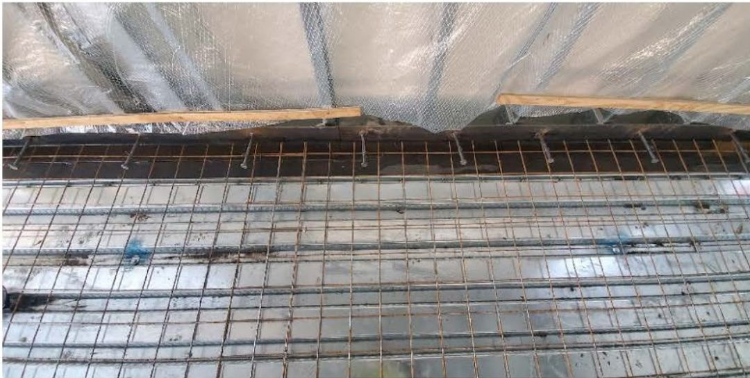
Image 2: Typical slab closure
