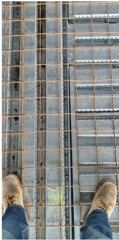
Image 5: Typical metal deck discontinuous edge
