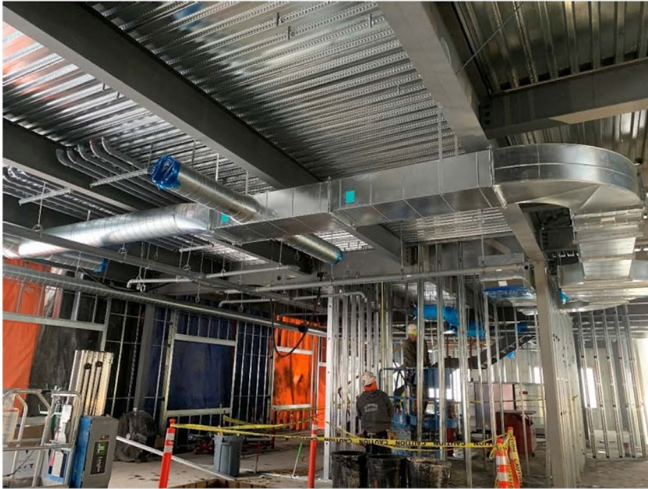
Figure 05: Ductwork and FCU install in Building 3B
