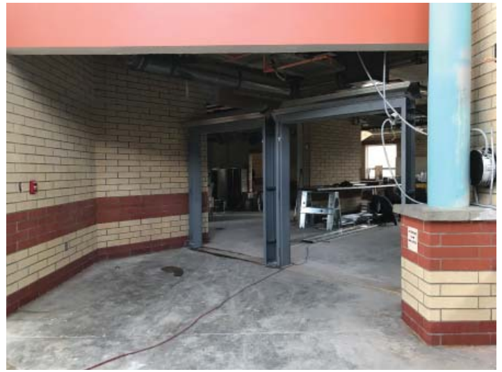
New main entry - steel door frames.
