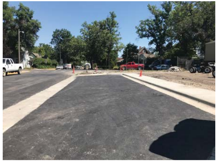
New asphalt, curb & gutter and sidewalk in place along Lamme St.
