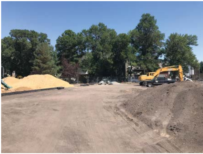
Regrading and soil amendment work in progress on the south end of the playground area.
