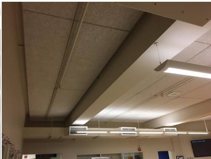
Tectum Ceiling - Multi-purpose Rm Complete
