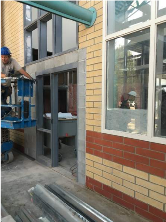
Lobby wall to be framed out with PLAM sill at window.
