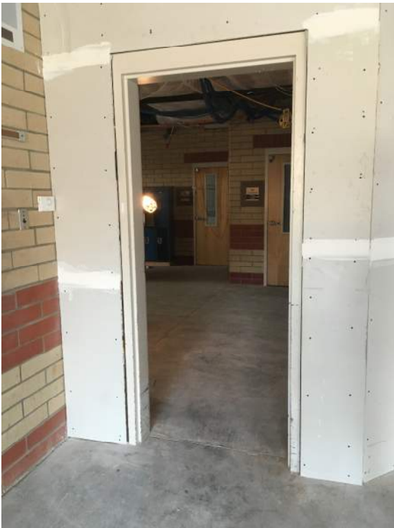
New framed wall at existing door.
