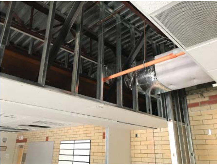
New support beam for operable classroom partition.
