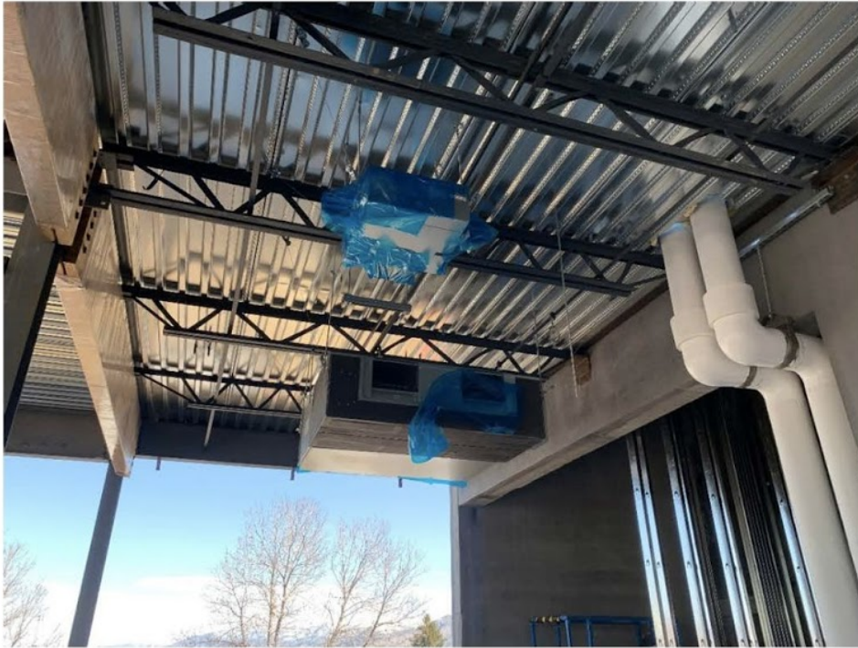
Figure 05: Replace protective covering on VRF fan coil unit.
