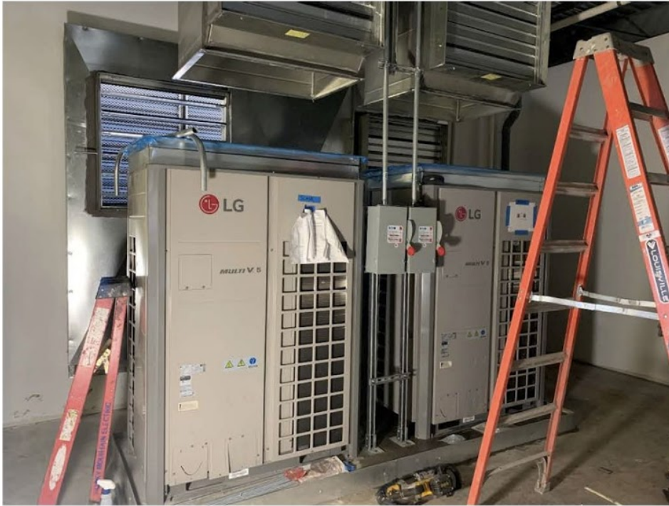
Figure 09: VRF ACCU installation in Mechanical Penthouse D302
