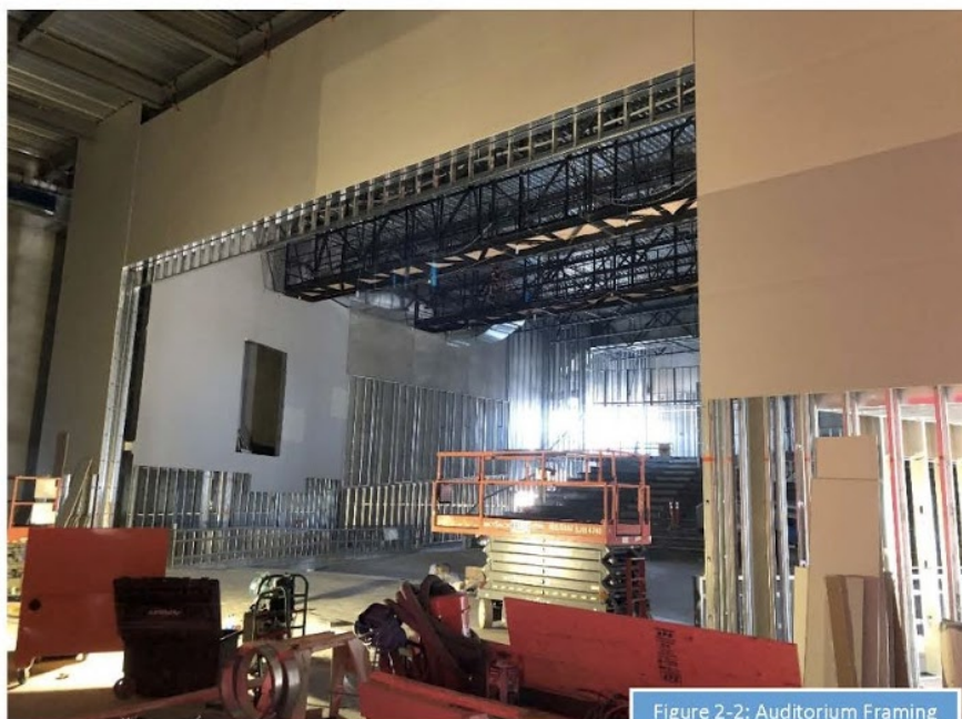
Figure 2-2: Auditorium Framing and Gypsum Wall Board
