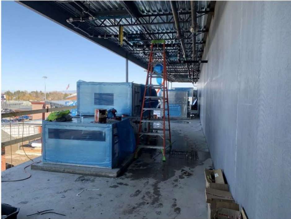
Figure 11: VAU-2, VAU-3, and AHU-1 installed in Mechanical Penthouse E303
