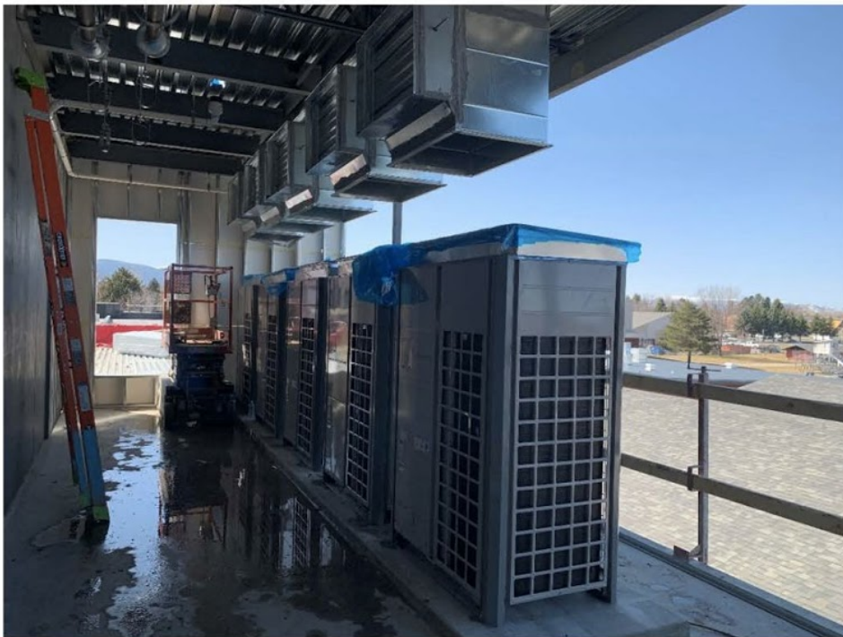
Figure 10: VRF ACCU installation in Mechanical Penthouse E303
