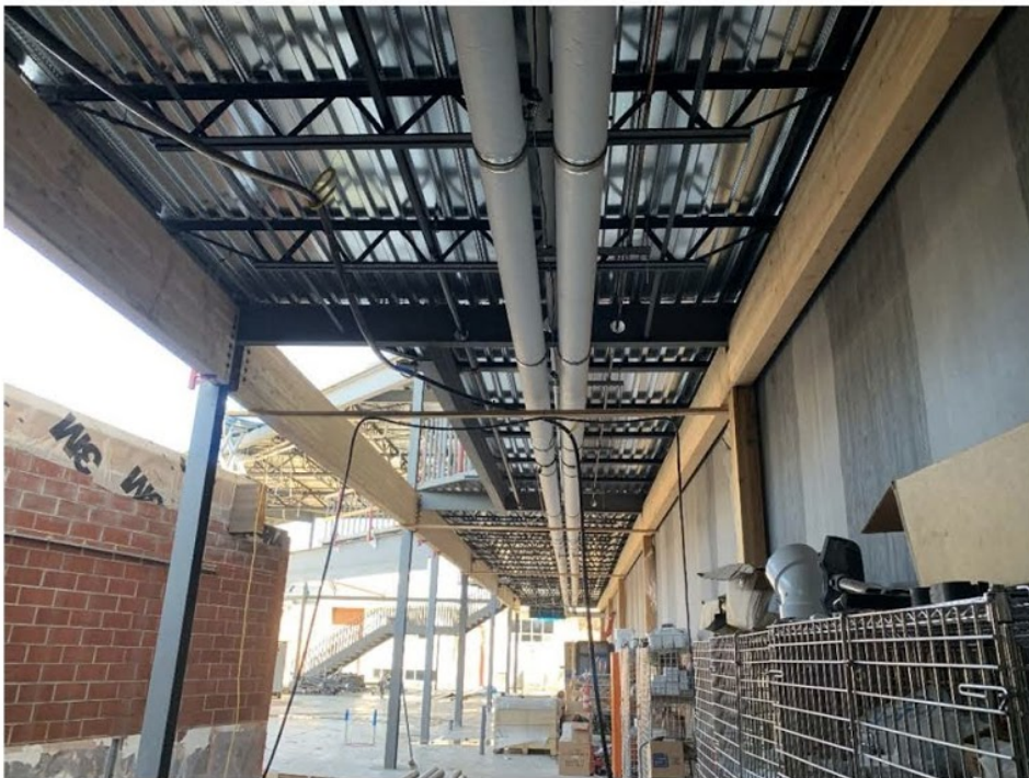
Figure 04: Hydronic Pipe installed in Building 2A.
