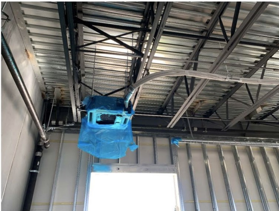
Figure 06: Replace protective covering on VRF fan coil unit.
