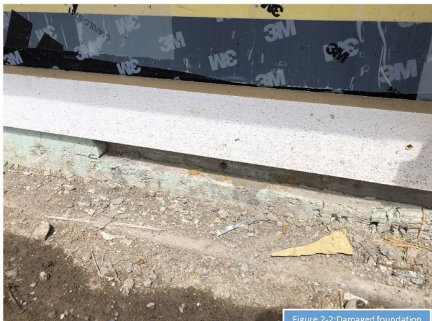
Figure 2-2:Damaged foundation Insulation At Classroom Wing
