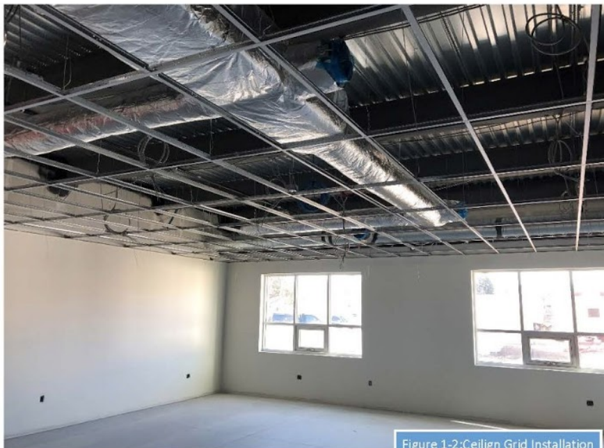
Figure 1-2: Ceilign Grid Installation at 3B
