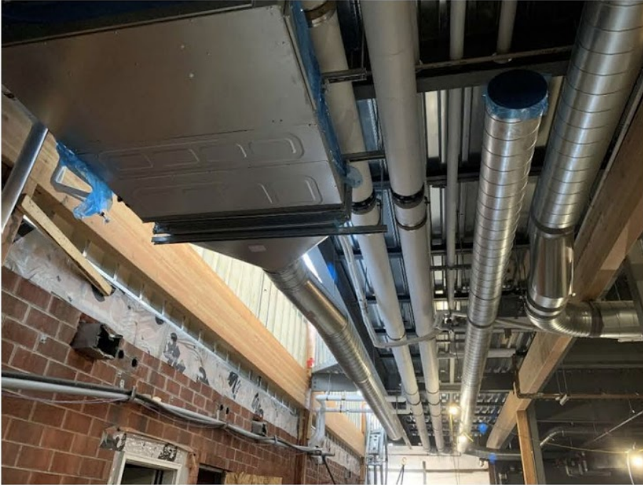
Figure 01: Ductwork and Hydronic Pipe in Building 3B.
