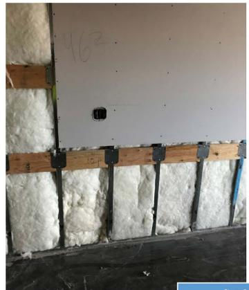
Figure 2-1: First floor 3B gypsum board installation
