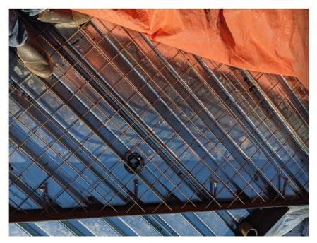
IMAGE 1: WELDED WIRE REINFORCING WITH CHAIRS. SLAB EDGE ANGLE WITH HEADED ANCHOR STUDS.
